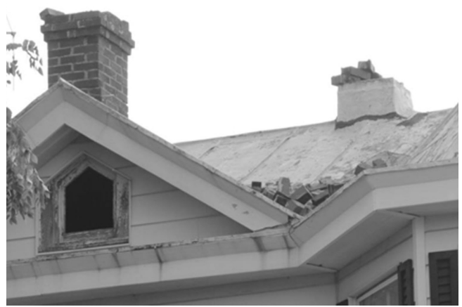
Damage from the 2011 earthquake in Mineral. Tom Leary photo.
